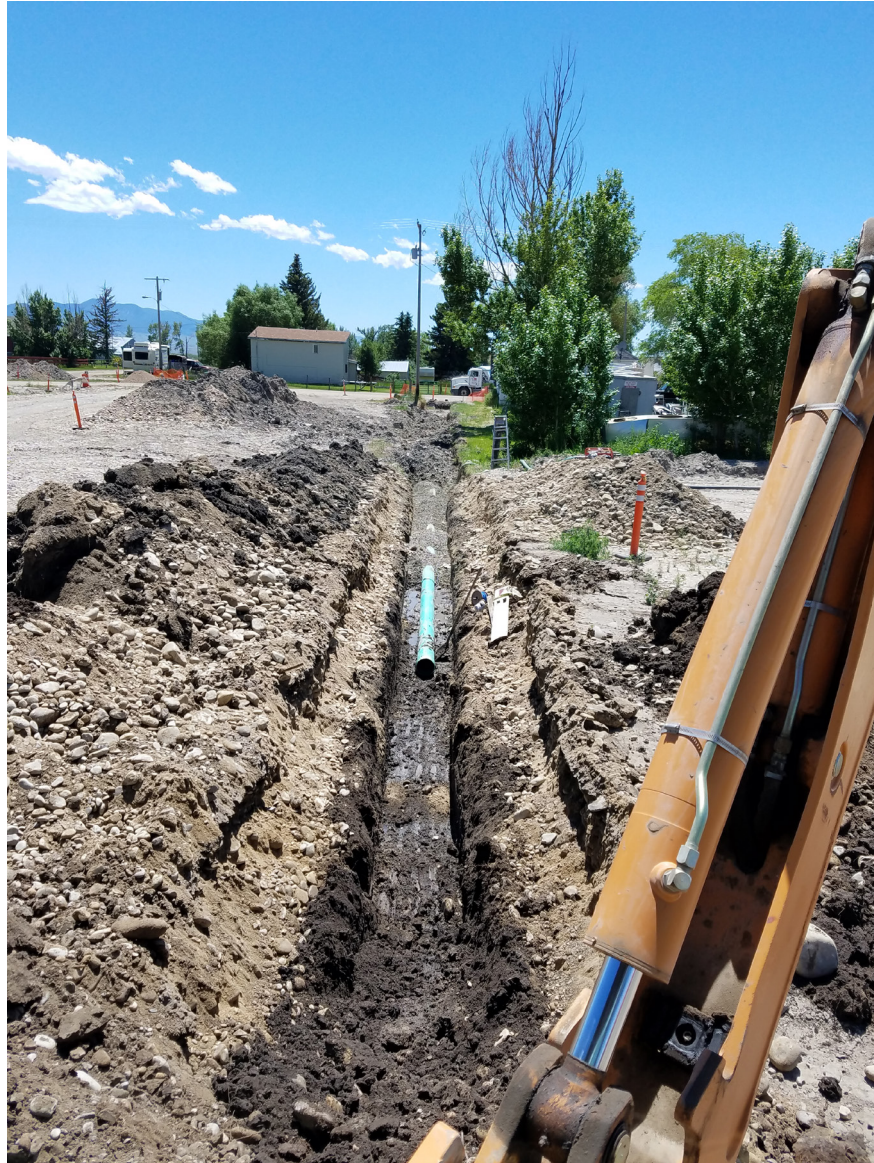
Figure 5 - Sewer System Extension on 9th Ave
