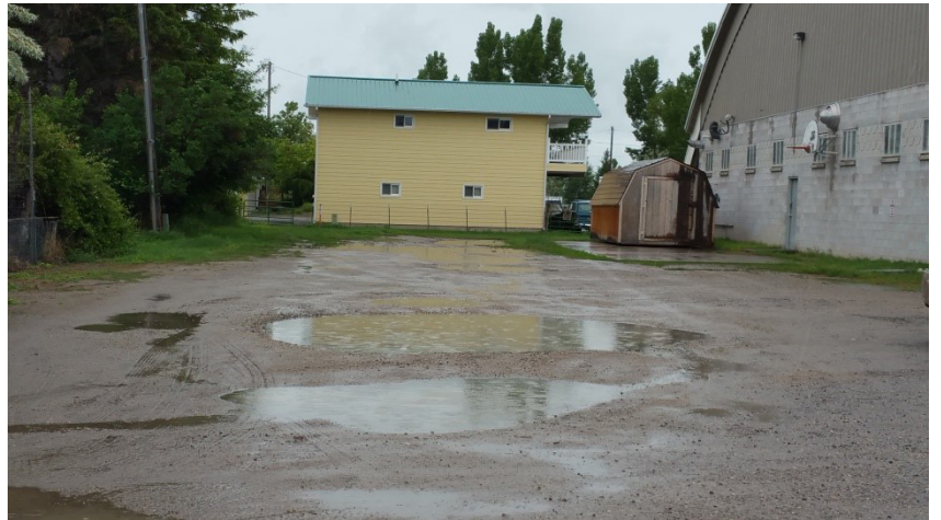
Figure 17 - Parking Lot Behind School Gym
